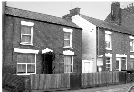
No. 44, West Street and neighbouring semi-detached houses
