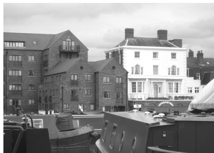
Below: Old and new buildings at Stourport
