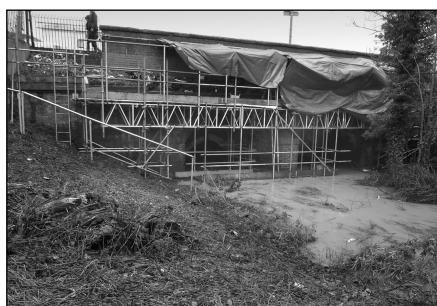
Below: Welcome clearance and landscaping undertaken by Network Rail.
