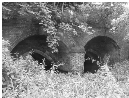
Above: Sycamore growing out of the Banbury bridge, showing the medieval arches of the original bridge beneath.
