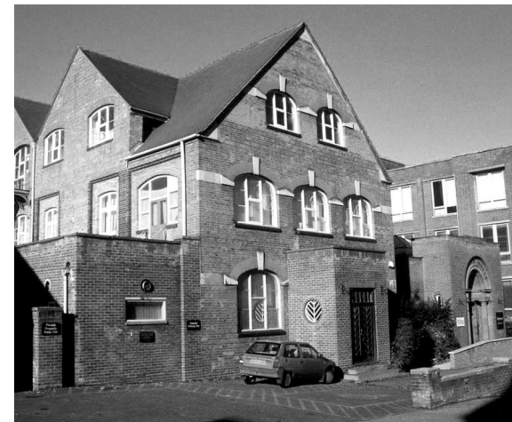
Spencer House before demolition
