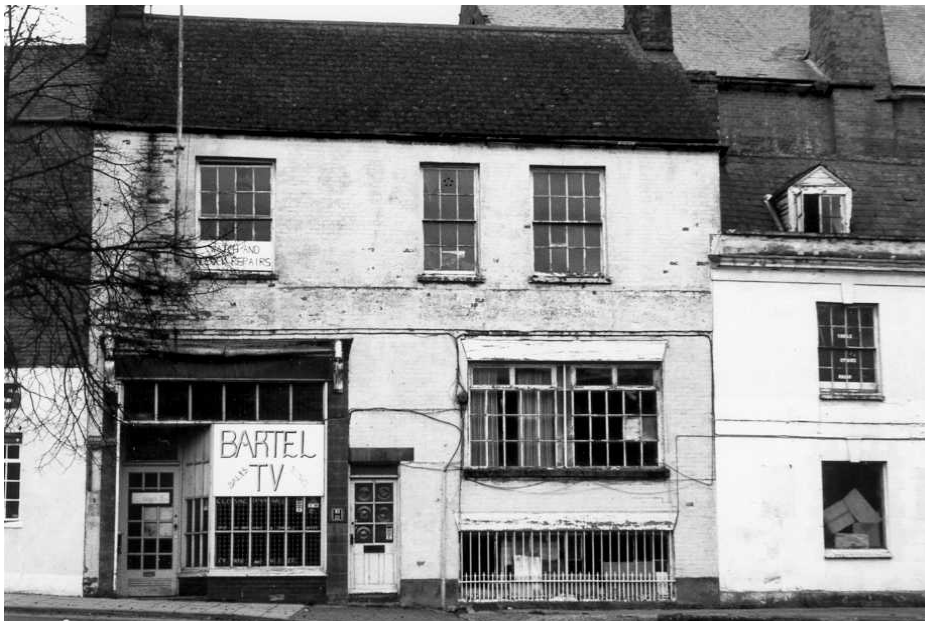
19 North Bar before demolition
